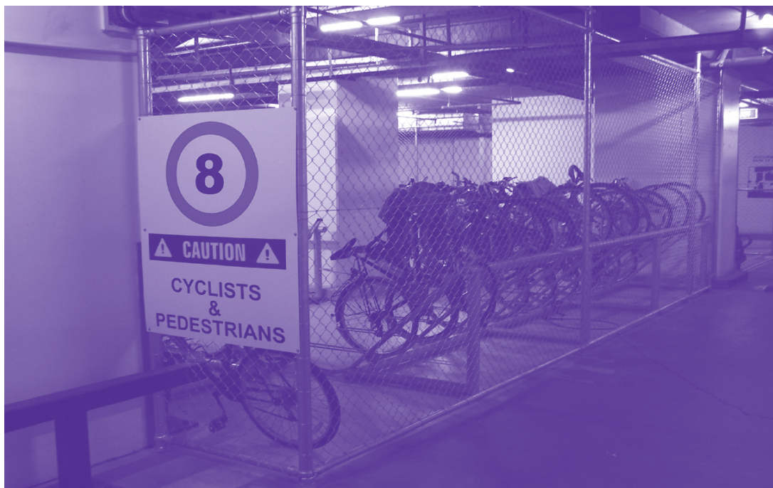
Figure 1: Accessing bicycle parking facilities via internal building lift - Brisbane Administrative Centre, Brisbane City Council
